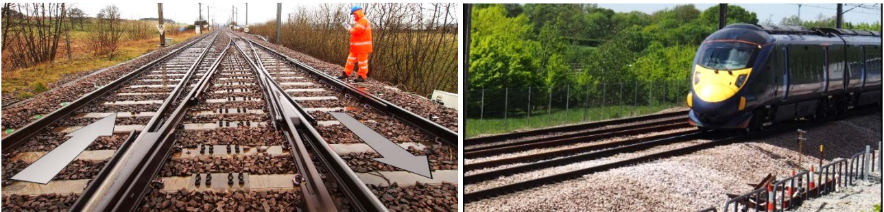
Fig.B1. USP field monitoring sites: (a) Wooden Gates S&C; and (b) Crissmill, HS1
